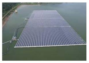
areas and solar panels are deployed in the Meghadrigedda water reservoir which reduced land-use issues. Also, it is saving water through mitigating evaporation and improving water security of the drinking water reservoir.
